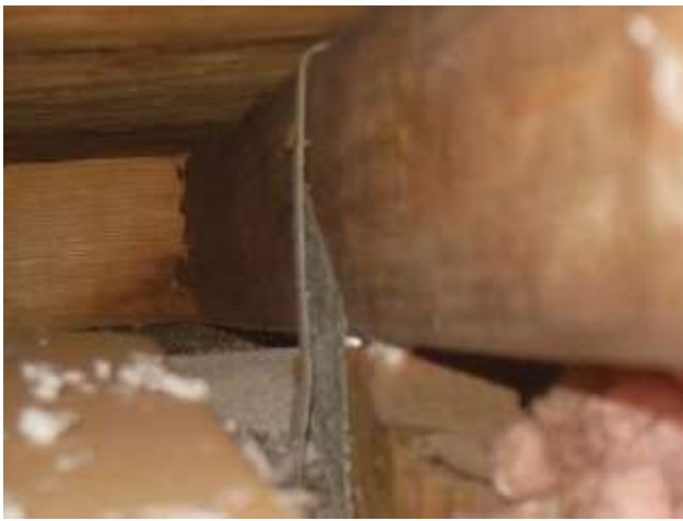
ROOF TO WALL - SINGLE WRAPS
