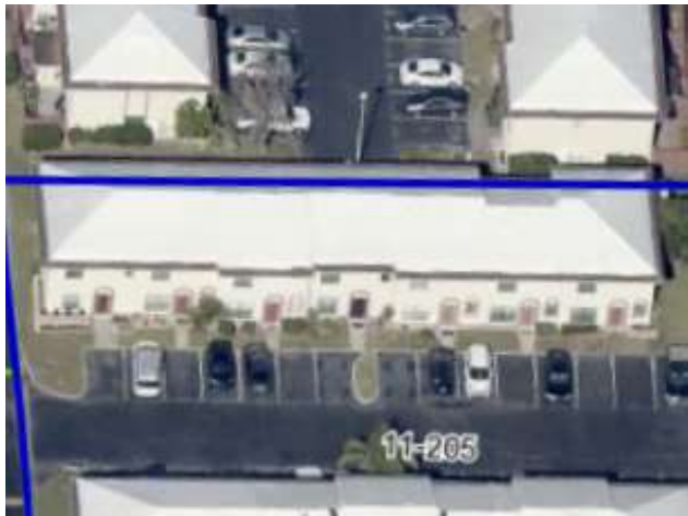
AERIAL VIEW SHOWING ALL HIP ROOF
