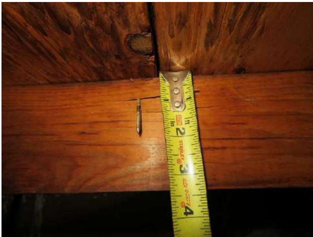
NAIL ATTACHMENT - 8D NAILS
