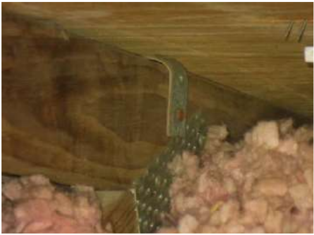
ROOF TO WALL - SINGLE WRAPS
